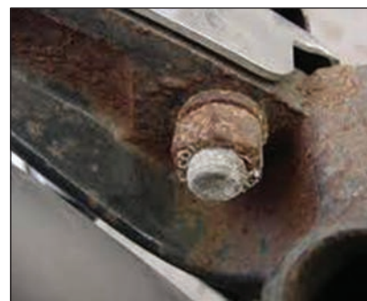
Figure 11. Rusty Bolts can cause PIM.
